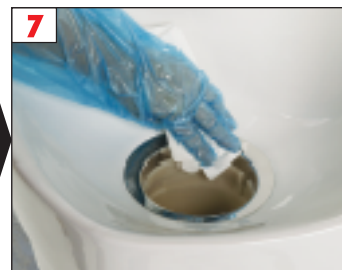
7 Wipe clean inner stainless steel rim
