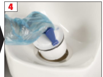
4 Lift cartridge and drain all free liquids
