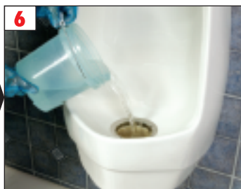
6 Flush housing with warm soapy water
