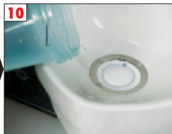
10 Fill cartridge with 1 quart or more of water until there are no air bubbles
