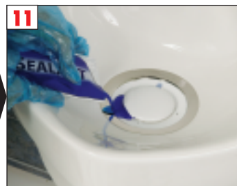
11 Add blue sealant and allow time to drain into cartridge
