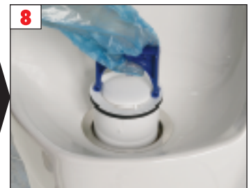
8 Insert new cartridge into housing
